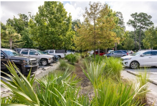
Bioswale planting in parking island manages stormwater and adds greenery.
