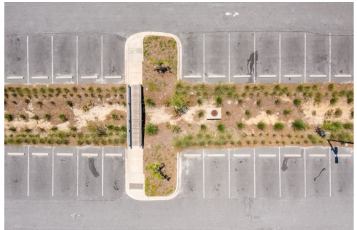
Newly planted rain garden improves both water quality and quantity management for the stormwater entering the parking lot.
