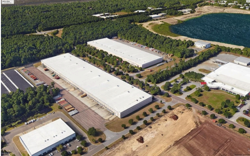
The industrial buildings are located close to the streetscape with a small amount of parking and drop off in the front, while the service area is located at the rear of the building.
