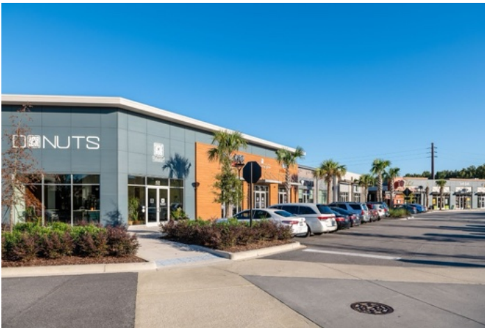
Foundation plantings enhance building facades by softening long stretches, highlighting architectural features, and improving the overall appearance.
