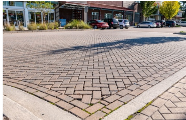
Pervious pavers manage runoff and improves site permeability.
