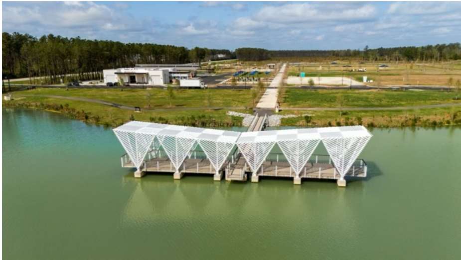
A retention pond with native vegetation supports stormwater and habitat.
