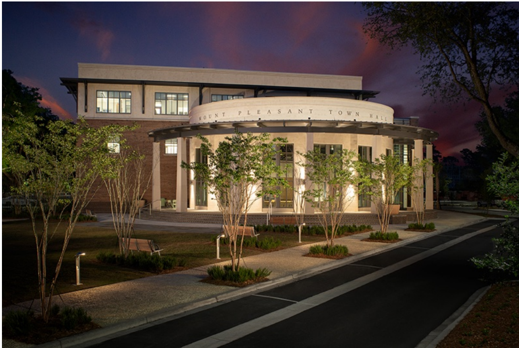
Simple exterior lighting illuminates parking, pathways, and building entrances.
